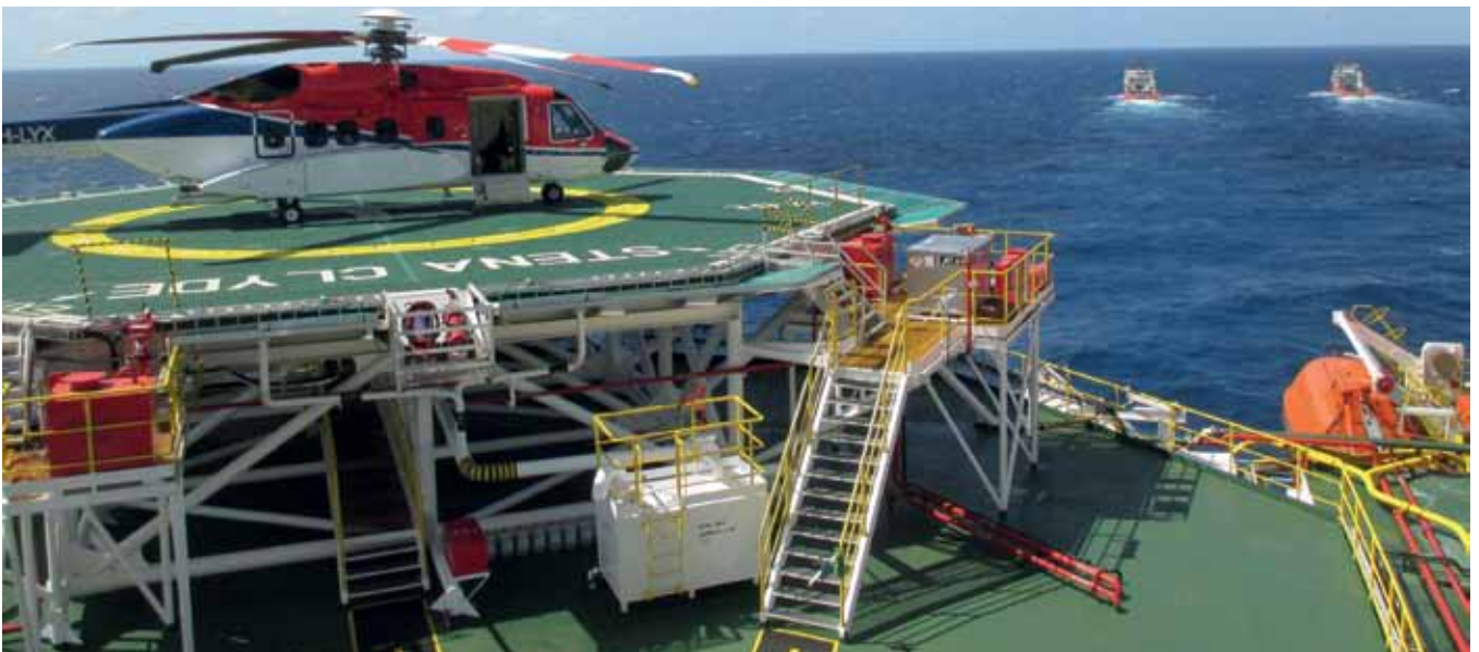
23 May 2015: Following the successful installation of the helideck and the earlier completion of its five-yearly special periodic survey (SPS), Stena Clyde leaves Singapore with a new lease of life
