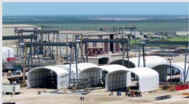
The specially designed domes for the outside assembly areas provides shelter from rain or shine to improve productivity
