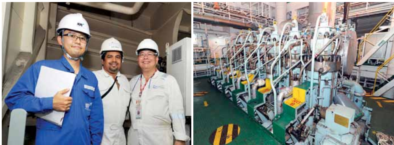
Dr Jerry Ng (right in the left photo), Founder and CEO, Blue Ocean Solutions (BOS), celebrating the successful installation of BOS Emulsified Fuel System on Diamond S Shipping's tanker, MT Agean Wave (main engine room seen in the right photo), with Diamond S Shipping and Korean Register of Shipping
